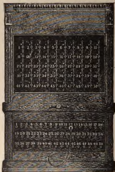
FIG. 212.—Annunciator-switchboard for hotel systems. By plugging a jack talking connections may be made between any room apparatus and the office.
